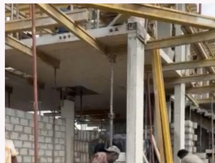
Preparation and formwork
