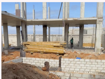
Structure under construction
