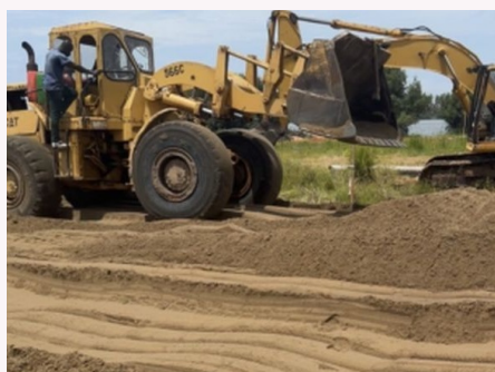
Equipment and materials on site
