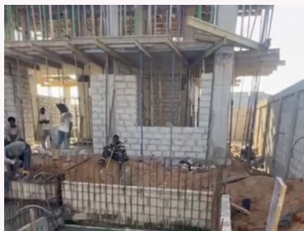
Reinforcement and structure
