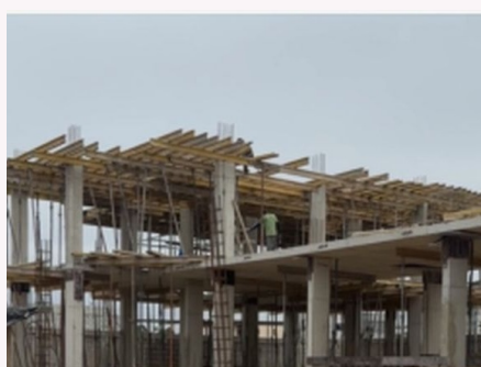
Structural works progress
