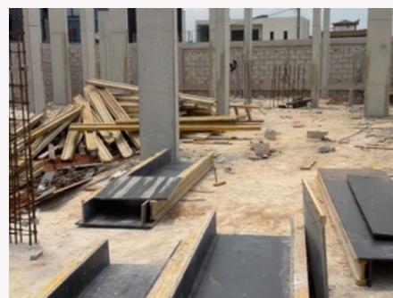
Formwork and preparation
